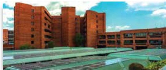
Kempton Civic Centre, Rooftop, South Africa
