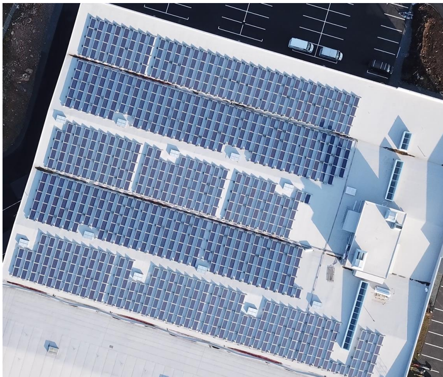
Location- Borlänge Capacity- 260KW
