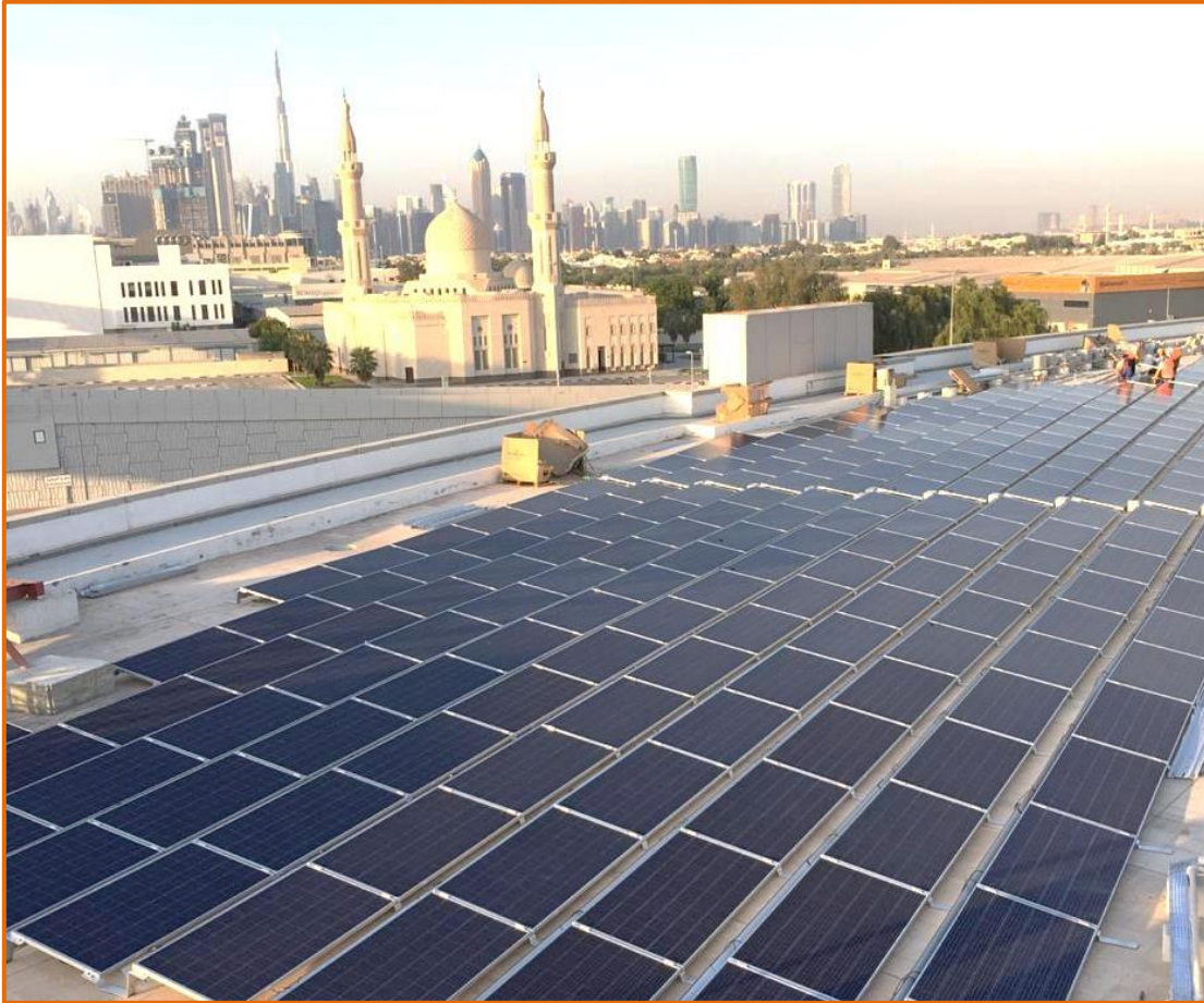
Location: The Curve Building, Sheikh Zayed Road, Al Quoz Capacity: 350 KW, 330 Wp Multi Crystalline PV Modules
